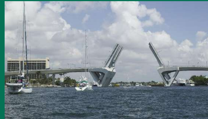
17 th Street Bridge, Ft. Lauderdale, Florida
