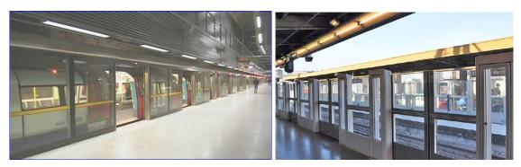
Platform Screen Doors can be designed for full coverage in underground stations, and partial coverage for surface and above-ground stations. (Source: Wikimedia Commons)
