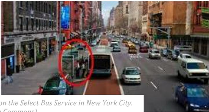
This type of treatment has a cost of approximately \$2 million per kilometre, a very low cost by any standard, as it simply involves painting red bus lanes that have been created by dedicating existing vehicle travel lanes, or by reducing on-street parking. This has
